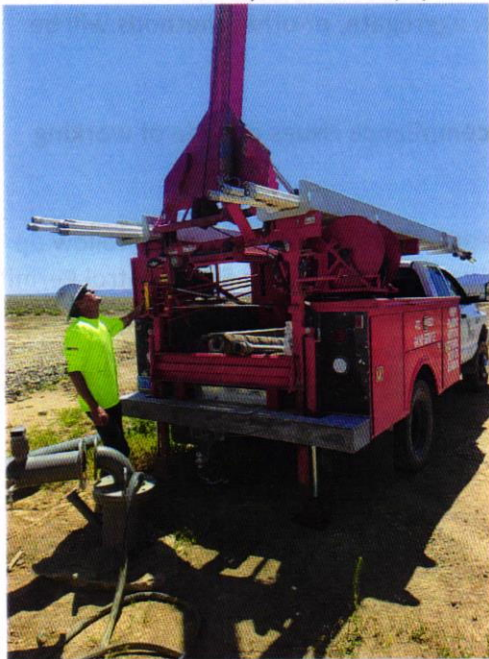
Saturday work (Crane to small)
