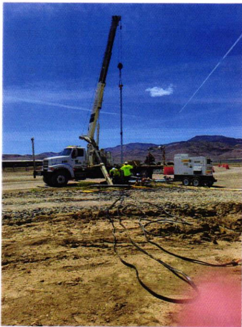
Friday work (up size the crane is working)
