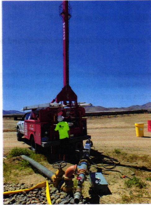
Saturday work (Crane to small)
