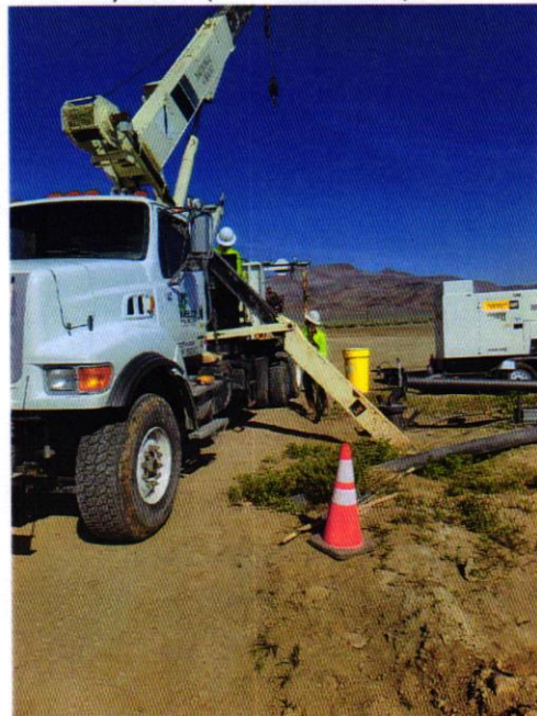
Friday work (up size the crane)
